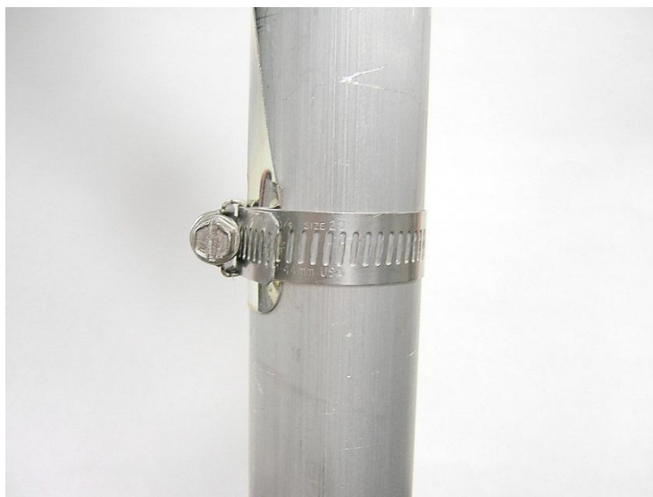
Figure 14 - Tower Bonding With Band Clamp
